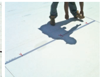
8' template bar marked with prescriptive grid measurements speeds layout
